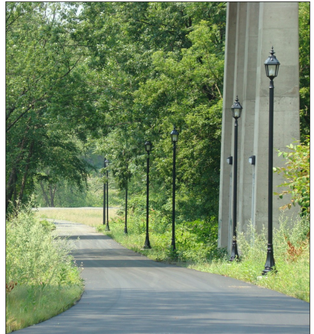
The Downtown Scranton Riverwalk under the Mulberry Street Bridge.
