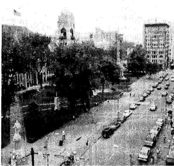
Figure 98: Contemporary view of Washington Avenue and Court House Square in downtown Scranton.
