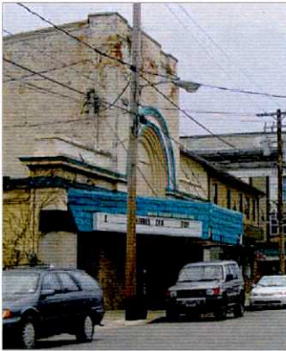
Vacant theatre in Olyphant Kise Straw & Kolodner photograph
