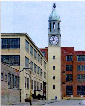
Adoptive re-use is planned for the former Scranton Lace factory. Kise Straw & Kolodner photograph
