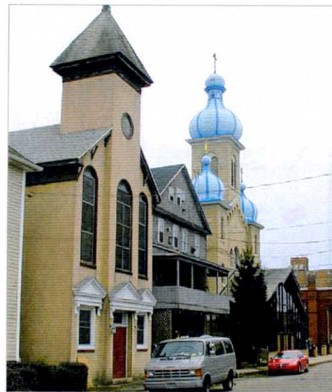
Former synagogue and All Saints Greek Orthodox Church, Olyphant Kise Straw & Kolodner photograph
