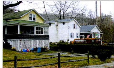
Laurel St. laborer housing with nearby PEI Cogeneration plant. Kise Straw & Kolodner photograph
